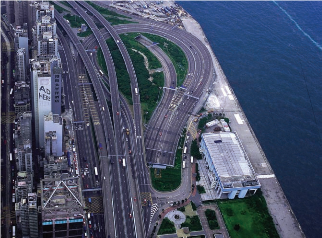
Western Harbour Crossing, HONG KONG
