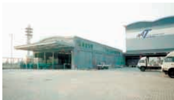
Western-By-Pass facility at Asia Airfreight Terminal
