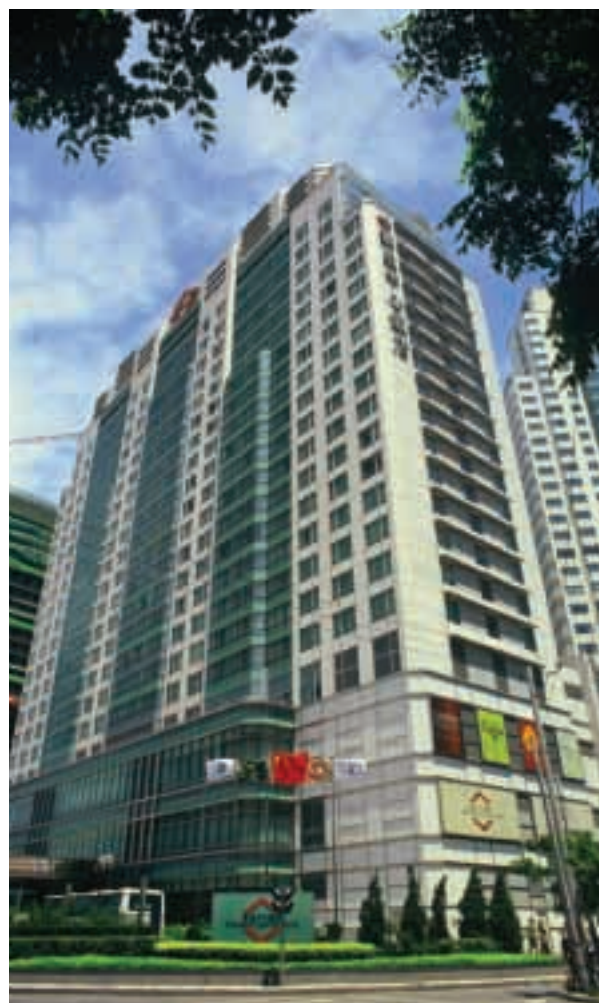
Beijing Kerry Centre Hotel, Beijing, PRC
