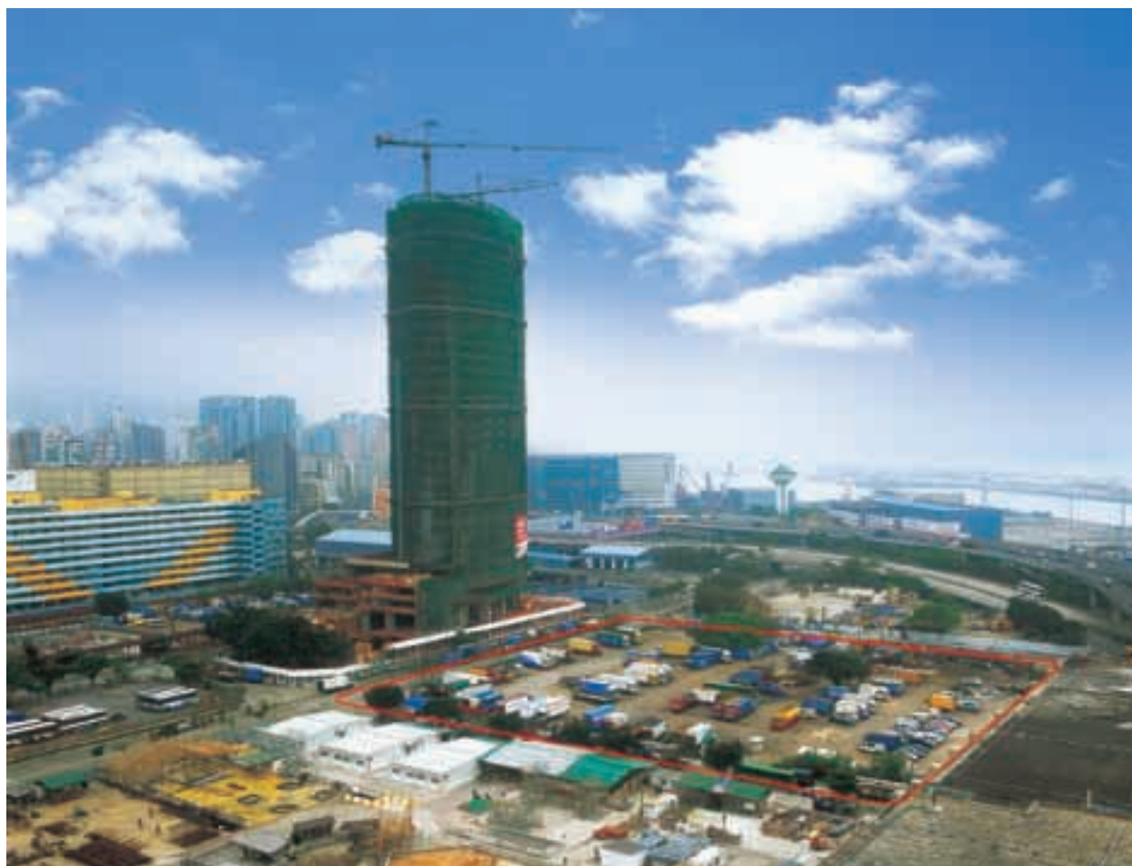
The construction of Enterprise Square 3 in progress with the site of Enterprise Square 5 in the foreground outlined in red in Kowloon Bay
